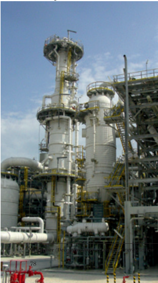
RasGas heat exchanger.
