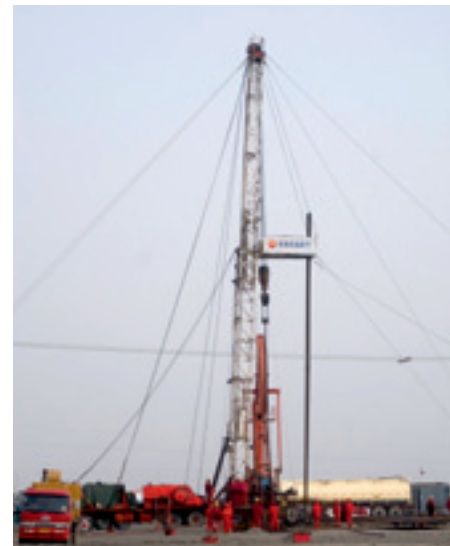
Petrochina oil pumping station in the Tuha oilfield outside of Turpan in the province of Xinjiang. Photo: Frans Schellekens
