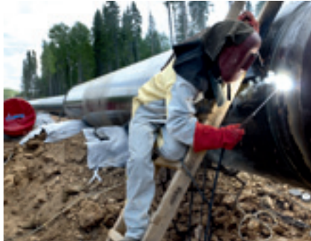
Working on Nord Stream. Photo: Wintershall
