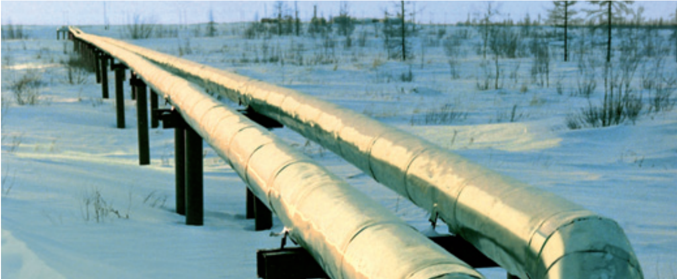
The new Nord Stream pipeline in progress. Photo: Wintershall
