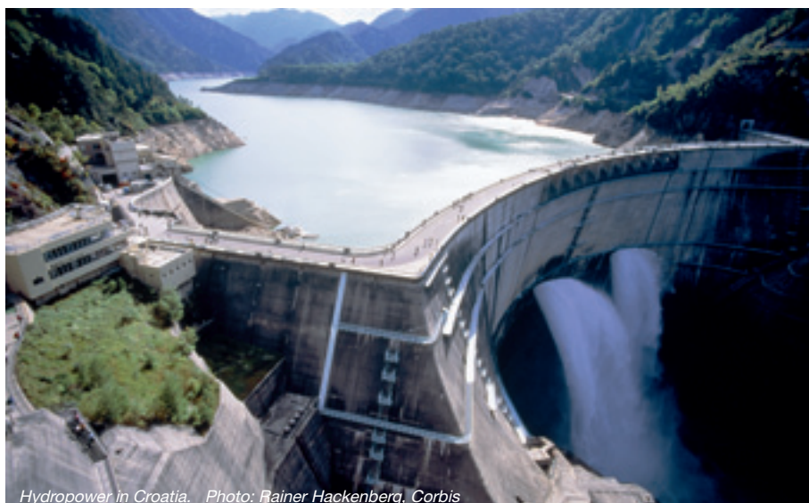
Hydropower in Croatia. Photo: Rainer Hackenberg, Corbis
