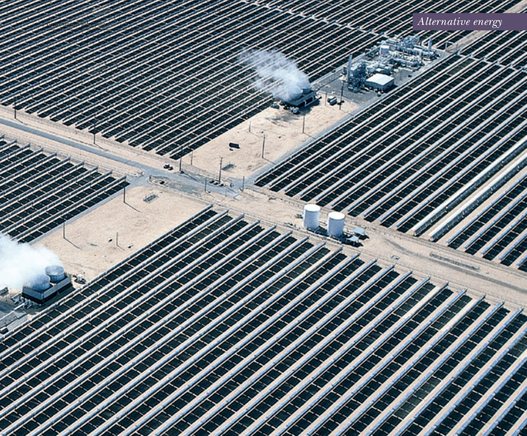
CSP-installation in Kramer Junction, California, in the Mojave desert.
