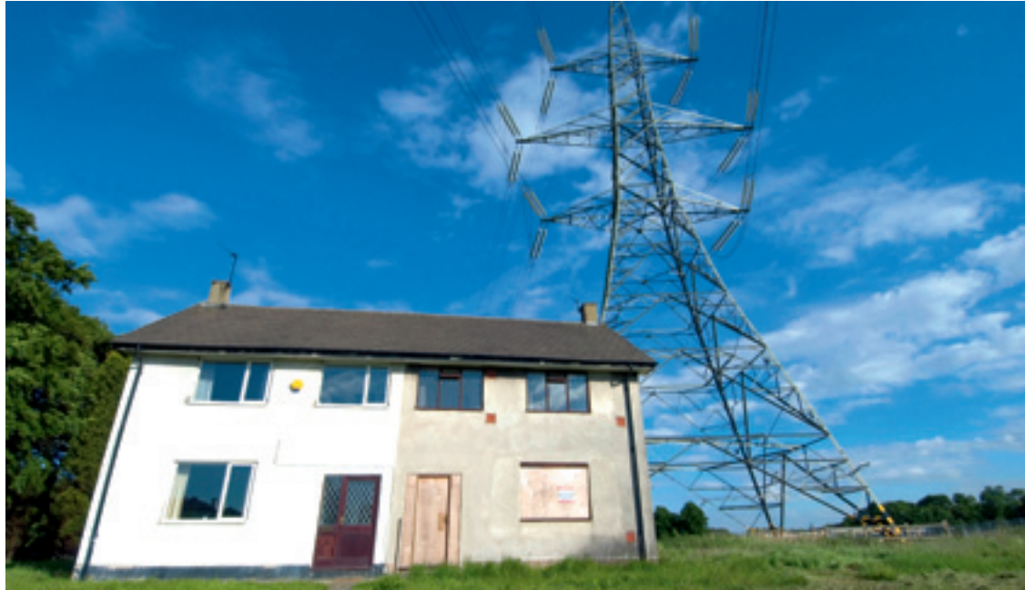
If the emphasis is placed on decentralized and small-scale electricity production, investments will mainly be needed in the medium and low voltage networks and to a lesser degree in the high voltage networks. Photo: Construction Photography/Corbis
