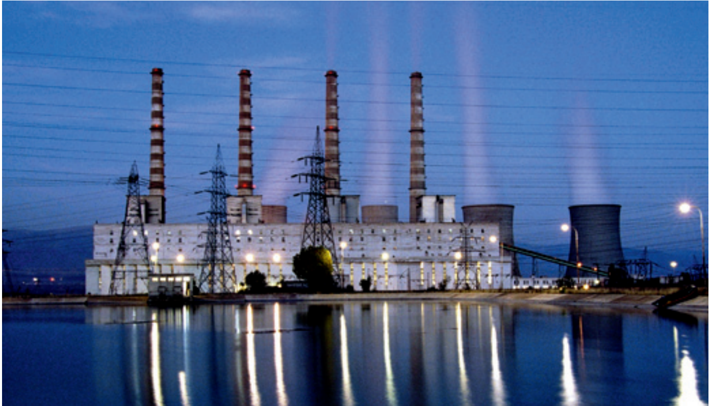
DEI's 550 MW Megalopoli lignite fired power station. Photo: Public Power Corporation S.A.
