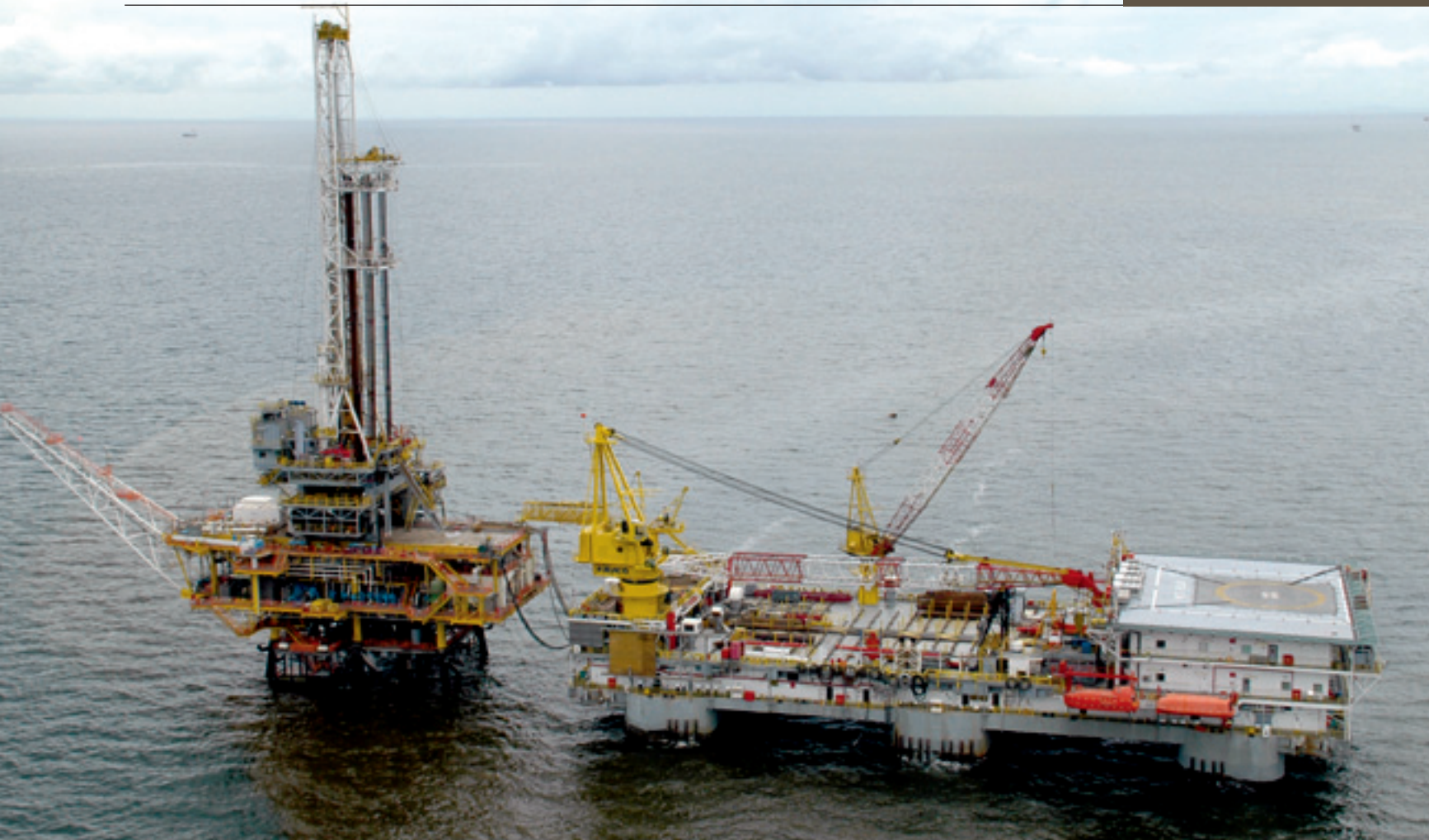
Unmanned smart field platform at Champion West, Brunei. Photo: Shell
