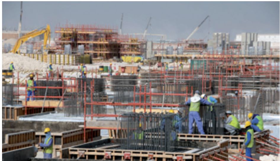
Construction of Pearl GTL. Photo: Shell
