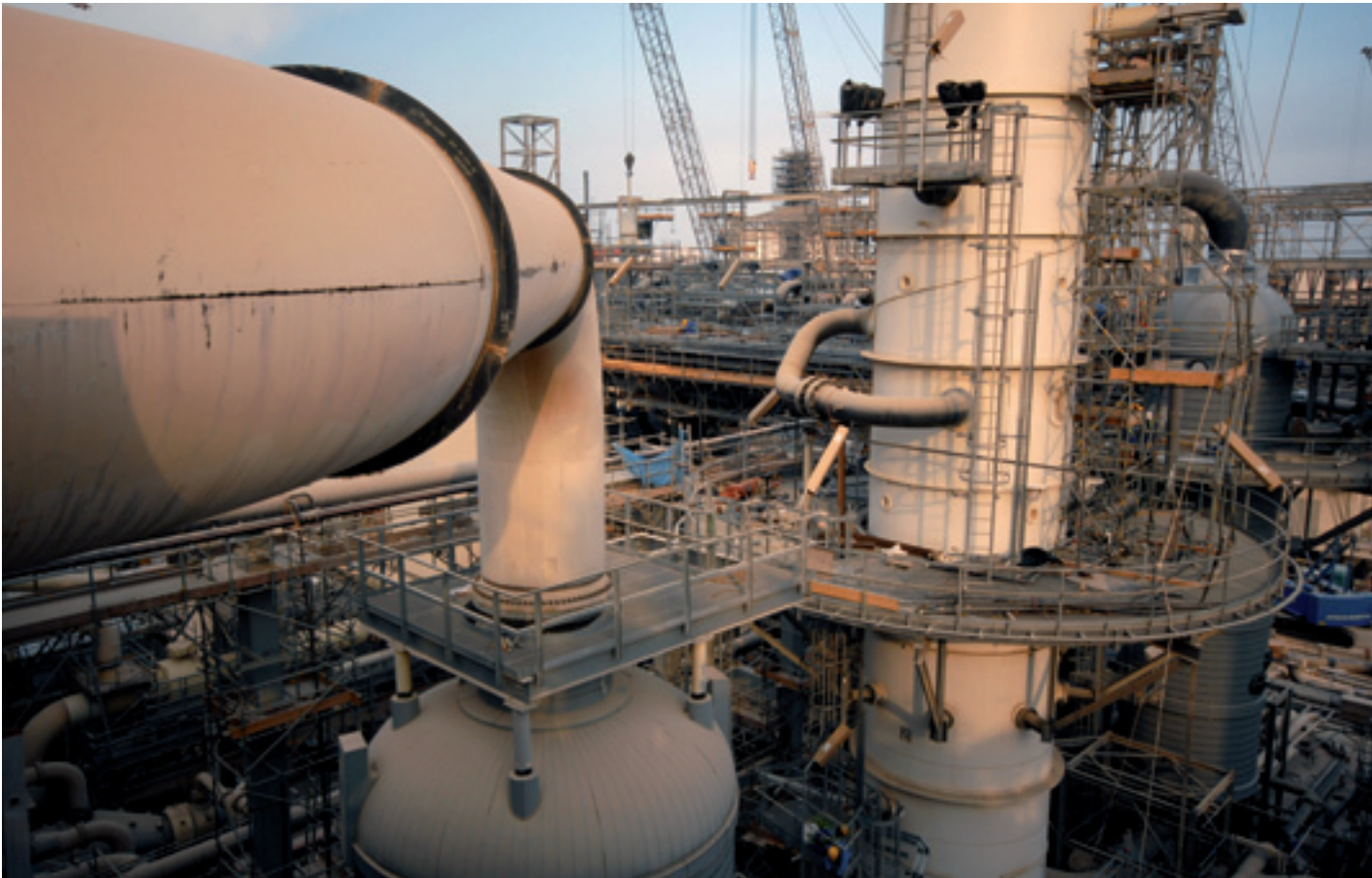
Construction at Qatargas 2, Doha, Qatar. Photo: Qatargas
