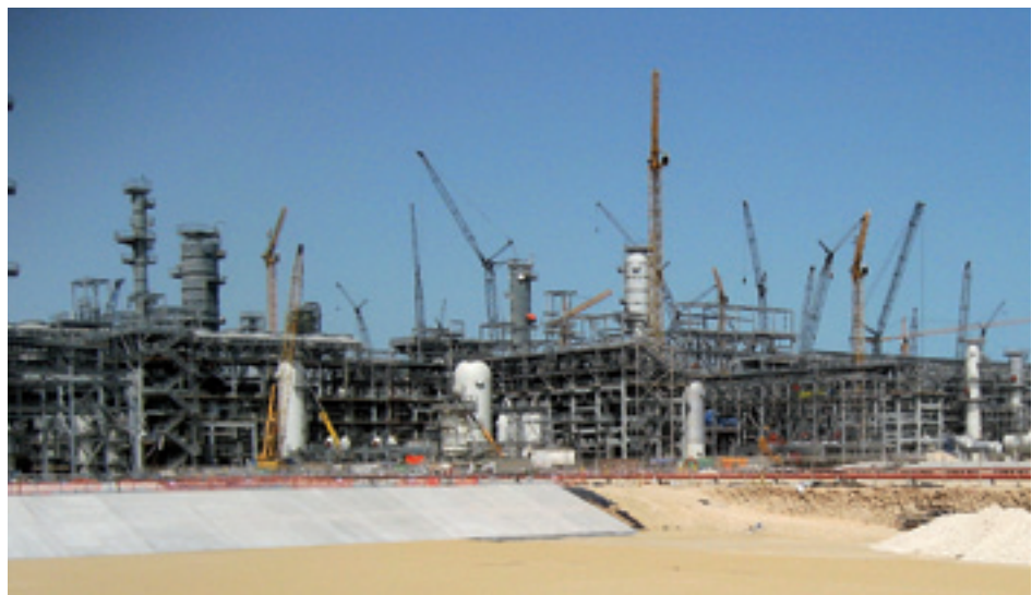
Mega-train construction at Qatargas 2. Photo: Alex Forbes
