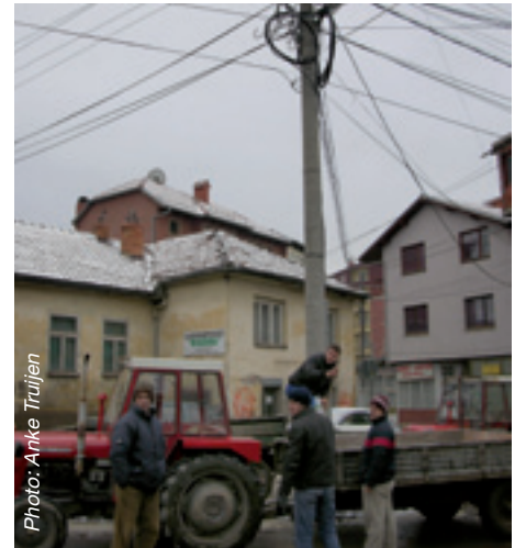
Photo: Anke Truijfen Power lines in the centre of Pristina.
