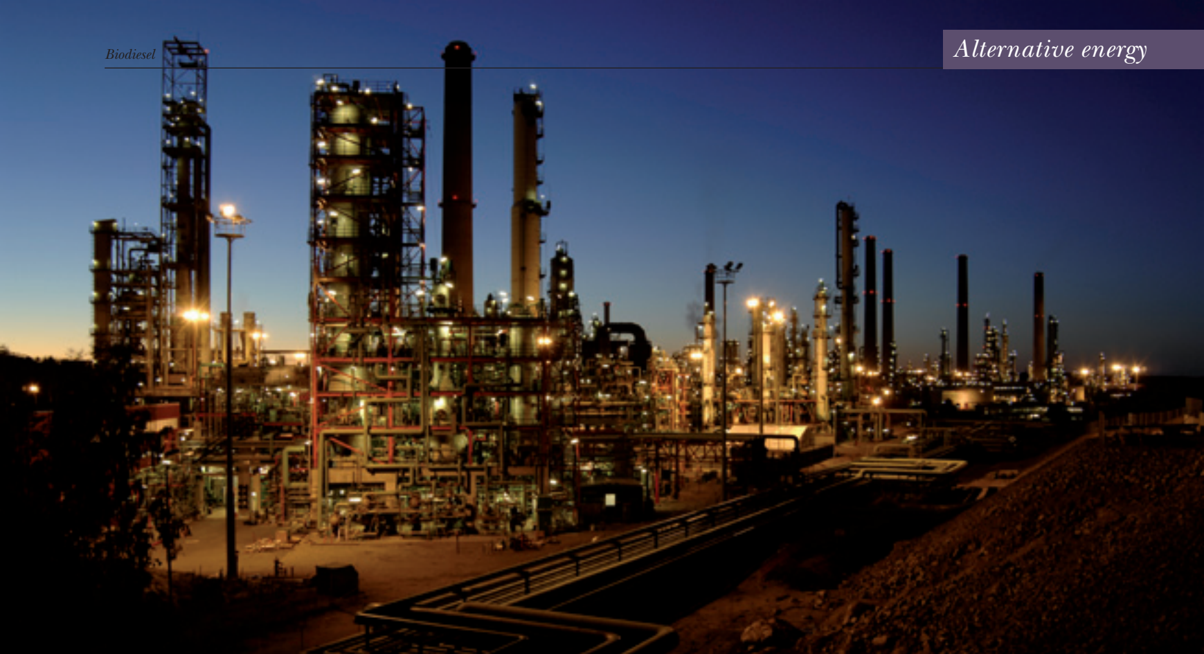
Biodiesel plant 1 in Porvoo, Finland. Erkki Ollikka/Neste Oil
