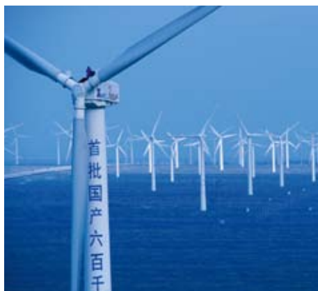
Dabancheng offshore wind farm in China. Photo: Bob Sacha/Corbis
