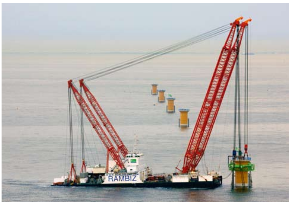
Special carrier “the Rambiz” lowers the foundations of the windmills on Thornbank. Photo: by C-Power
