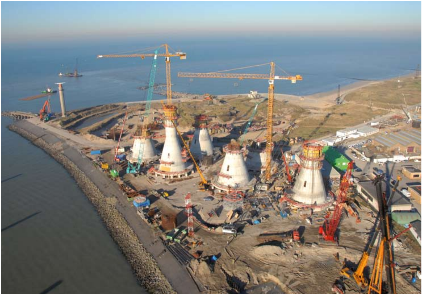
The "Half Moon" construction site in Ostend. Photo: by C-Power
