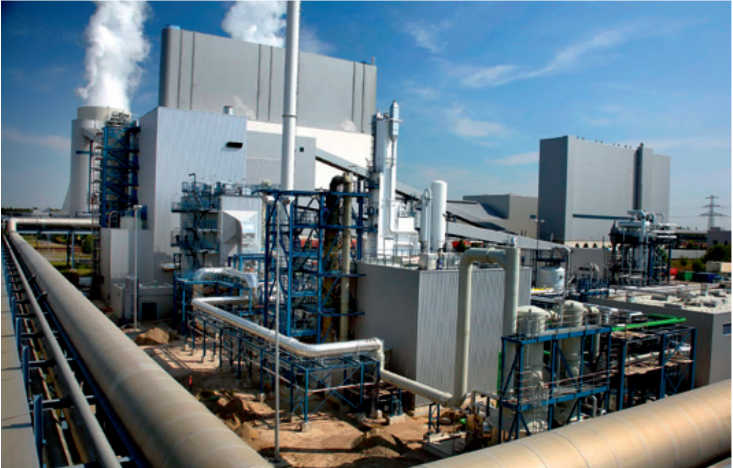
Oxyfuel carbon capture plant at Schwarze Pumpe Photo: Vattenfall
