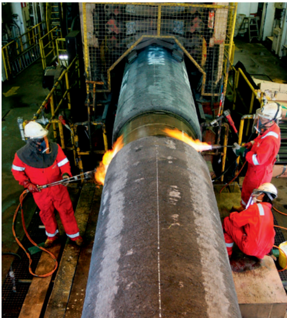
Pipelaying vessel Acergy Piper off Norway. Photo: Scott Barbour/Getty
