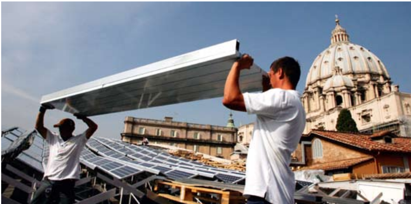
Solar power panels are placed on the roof of the Nervi-Paul VI Hall, in the Vatican. Photo: Giuseppe Giglia/EPA
