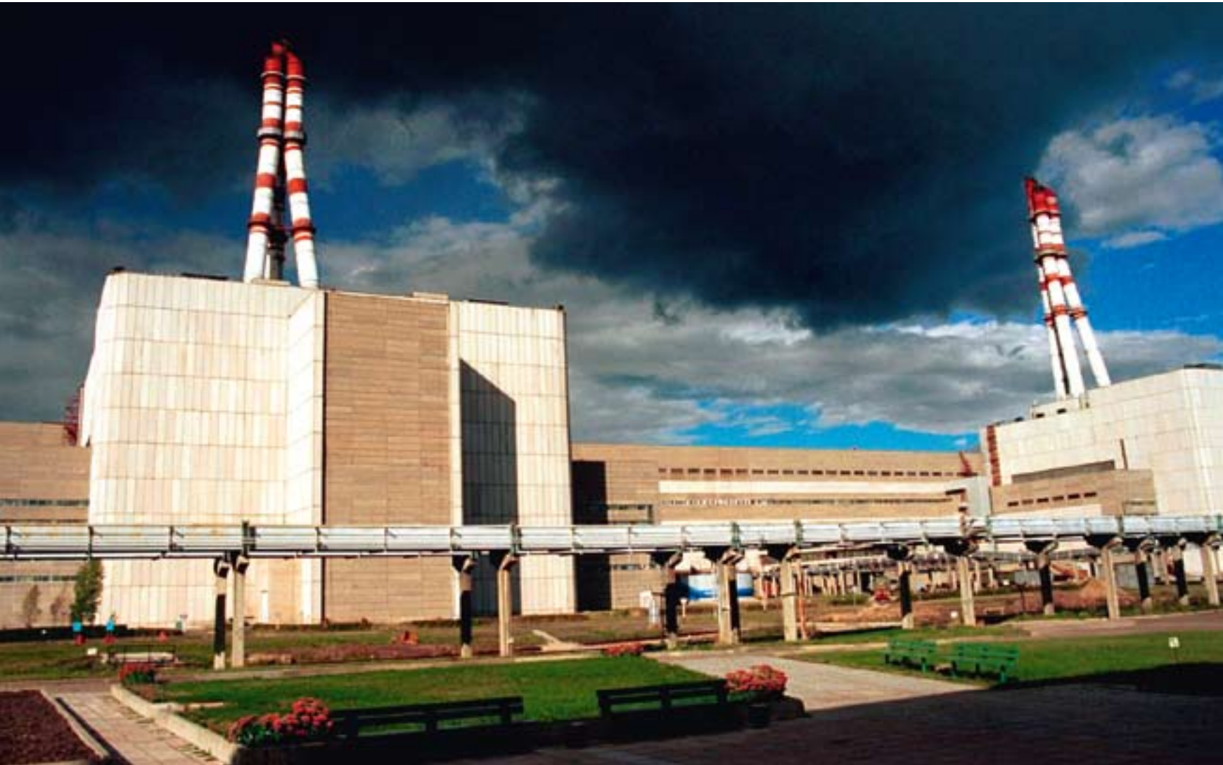
The Ignalina nuclear power plant in Lithuania. Photo: EPA/AFI
