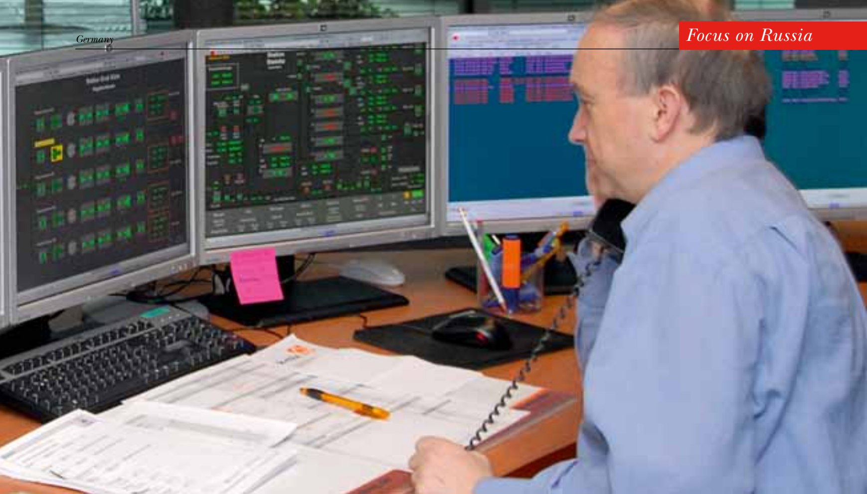
Control room of VNG. Photo: Bodo Tiedemann
