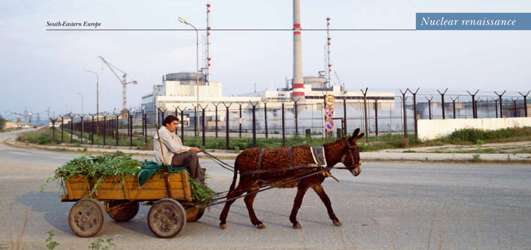
Nuclear Power Plant in Kozloduy, Bulgaria. Photo: Robert Wallis/Corbis
