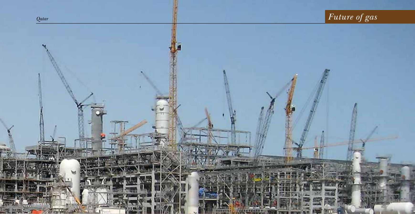
Construction at Qatargas 2, Doha, Qatar. Photo by: Qatargas
