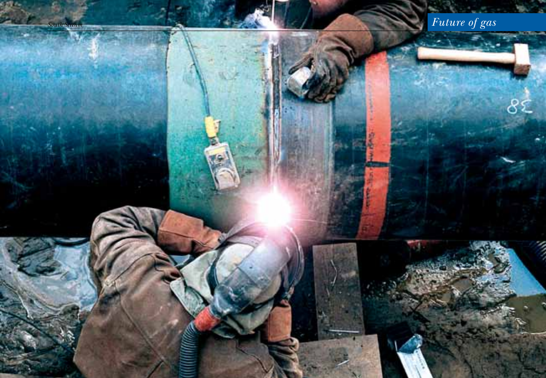
Workers welding two pipeline sections together. Photo: Goedan/laif/Corbis
